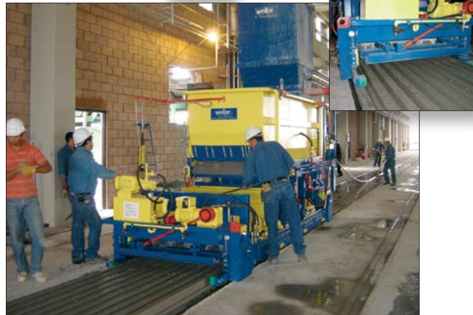
betonieren placing of concrete
