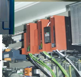
Electronic SEW servo controllers for precision synchronization of motor speeds, torques & drives.
