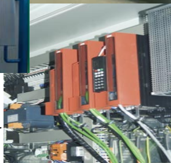
Electronic SEW servo controllers for precision synchronization of motor speeds, torques & drives.
